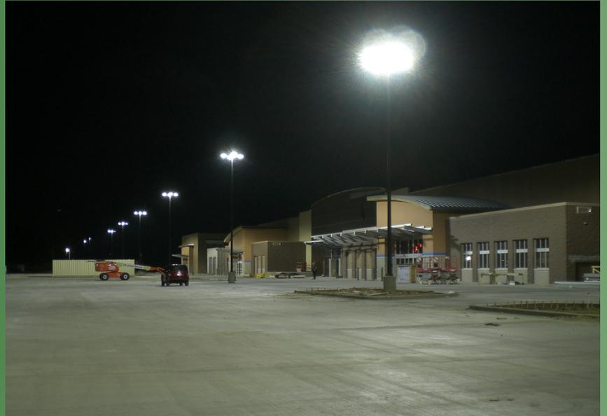
“Typical concrete has a higher reflectance value than asphalt, along with a smoother, more reflective texture. The higher reflectance values from concrete play as much of a role in the visibility and apparent brightness of the site as the lighting.”
